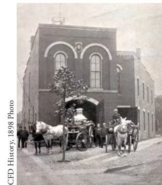
Station No. 6 - 1898 Photo
