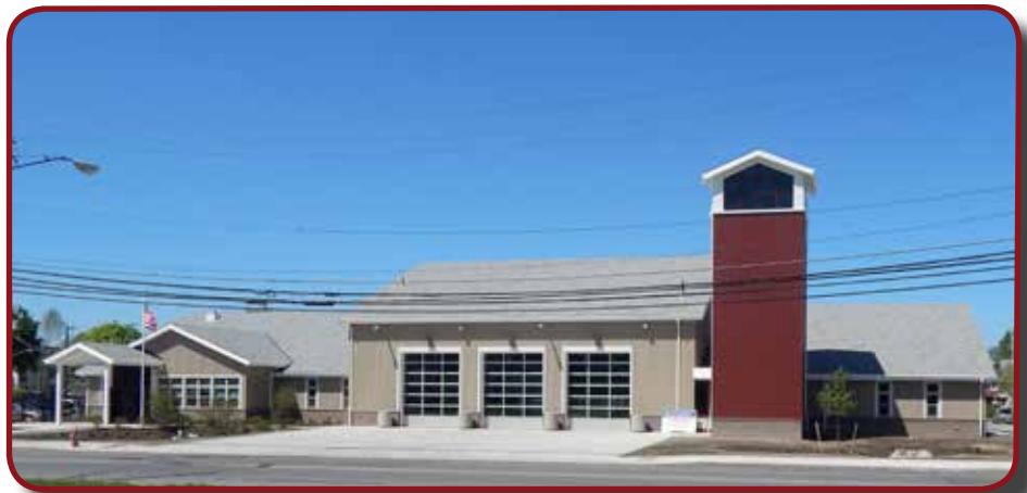
New Station No. 36 at 3553 E. 131st Street
