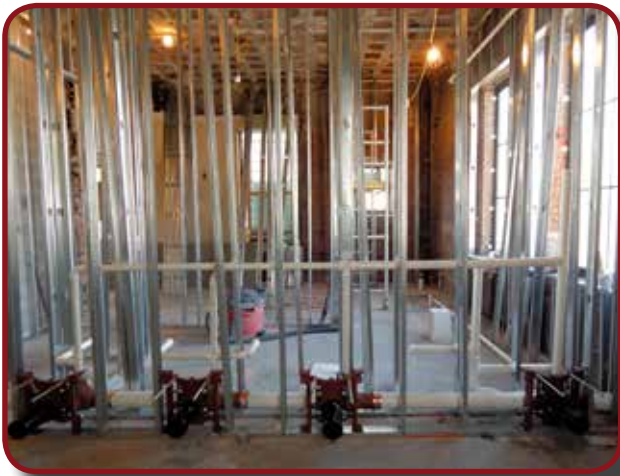
New bathroom construction
