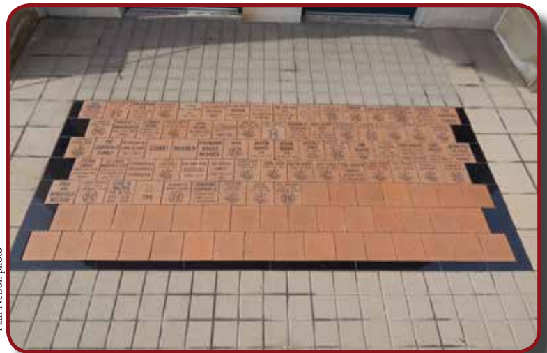
First batch of pavers in place
