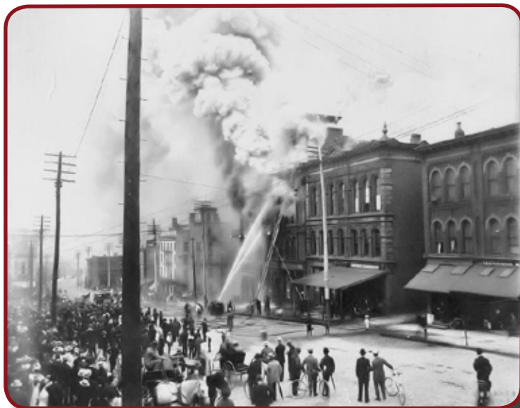
The 65-ft ladder thrown to the roof
