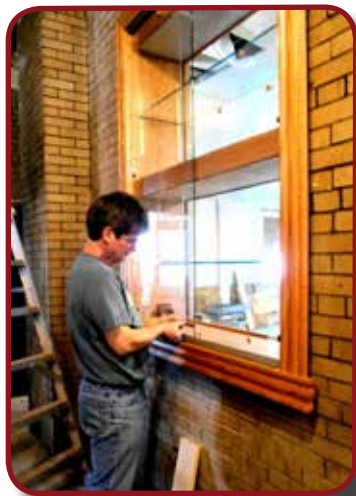
Tim Clark installing window
