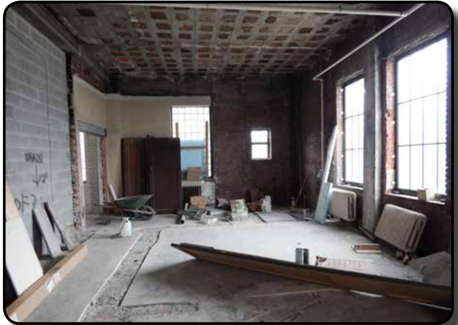
Second floor bathroom is one of the projects to be finished
