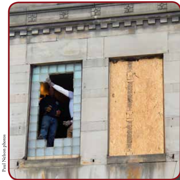
Removing the glass blocks
