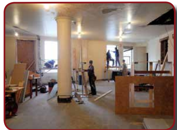
Getting ready to install temporary closures
