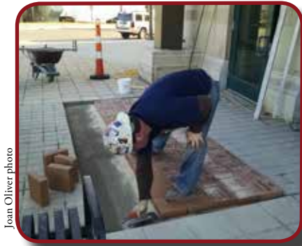
Initial Paver Installation
