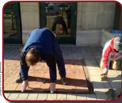
Granite Border Installation
