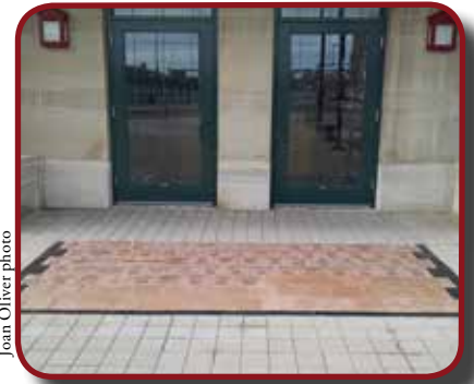
Finished Pavers in Place
