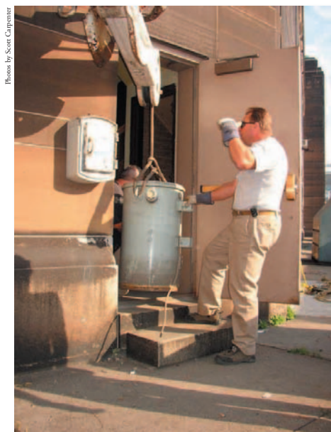
CPP removed old and unused transformers from the electrical vault.
