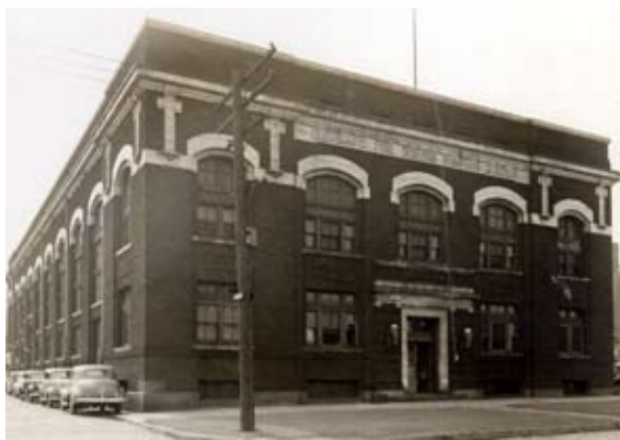
High Pressure Pumping Station shown in 1940 CFD Archives photo
