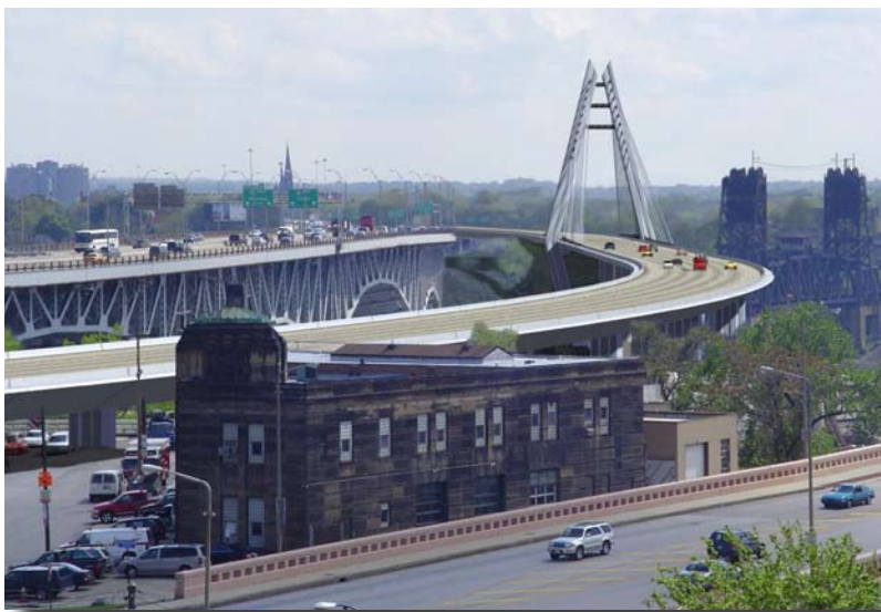
After looking at several options for bridge designs, ODOT is proposing a single tower cable-stay bridge. This photo shows how the bridge and the road will look with our building in the foreground. What's not shown is the on-ramp from Ontario. The on-ramp will be next to the bridge, adding a fifth lane to the system. It is not yet clear how the on-ramp impacts the site.
