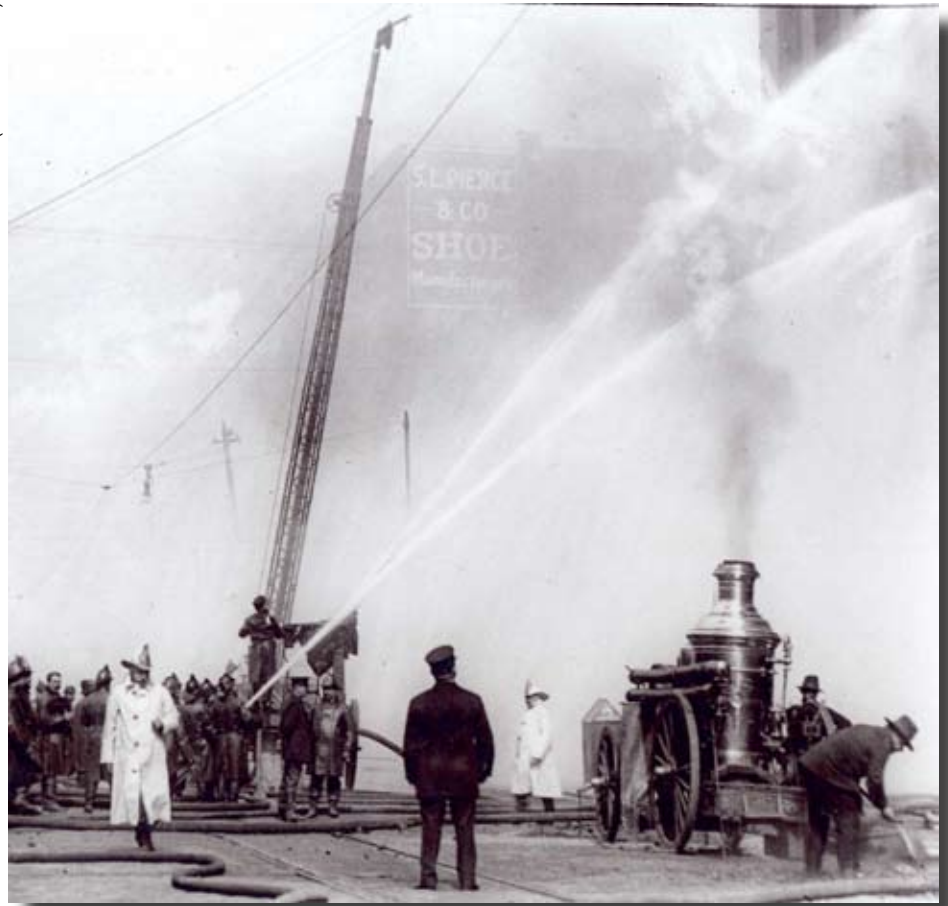
Tower No. 1 operating on W. 3rd Street before wall collapse
