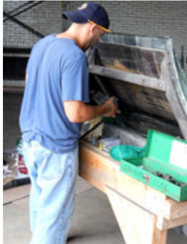
PETE SIMON, ENGINE 11, INSTALLING FIRE ALARM SYSTEM
