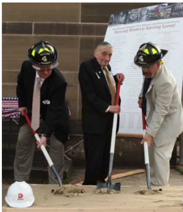
John Zangerle, Sam Miller, and Dan Hayden take up their shovels at the Groundbreaking.
