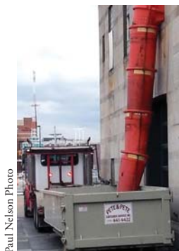
Debris was thrown through the window to a dumpster below
