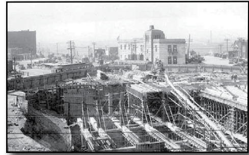
Railroad cut and area around Station 28 finished - 1930
