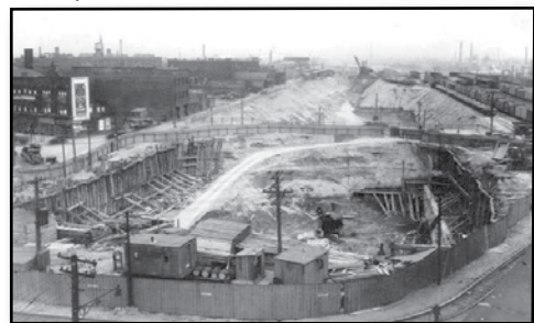
Railroad cut at Central Viaduct Roadway - 1928
