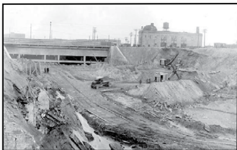
Looking south from Eagle St. toward Central Ave. - 1929
