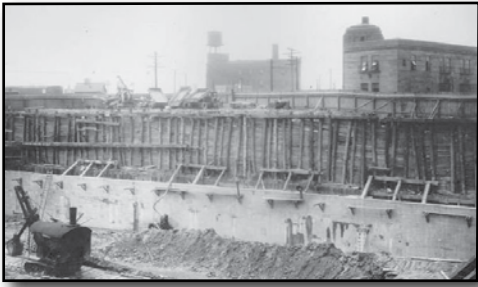
Retaining wall below Central Ave. - 1928/1929
