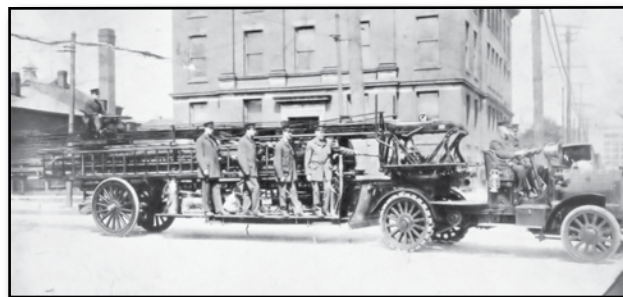
Ladder 7 1913 Peerless tractor 1901 Rumsey Kaiser 75-ft aerial ladder with air hoist
