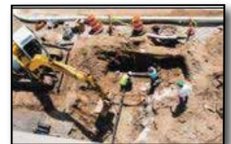
Water line installed June 2013
