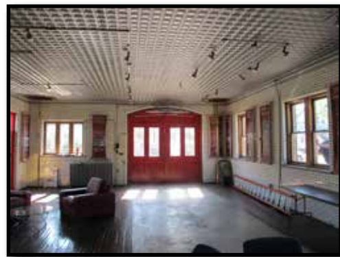
Tin ceiling in restored Station 3
