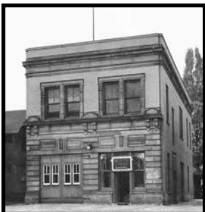
Fire Station 34, 12010 Ashbury Ave.
