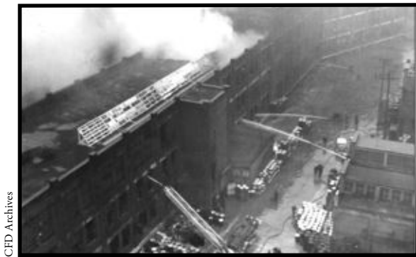
Building 21 where fire originated
