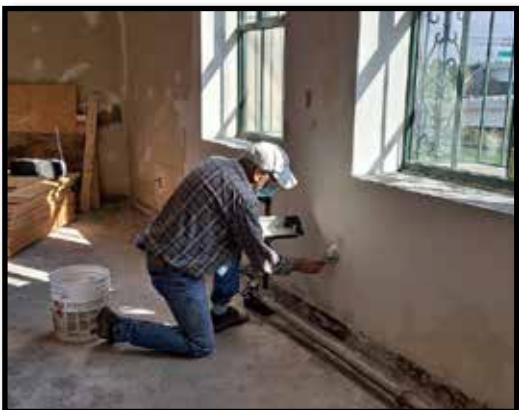
Richard Lash busy plastering dormitory walls
