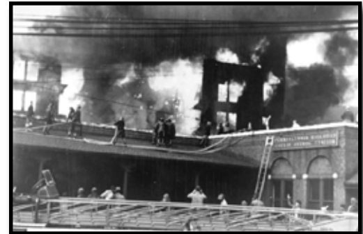
Companies working on roof of Pennsylvania RR station
