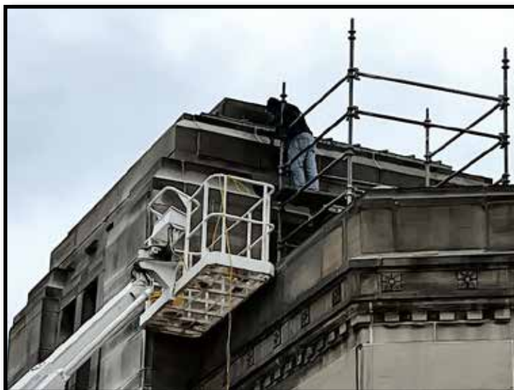
Coon Restoration Starts Work on Building Repairs
