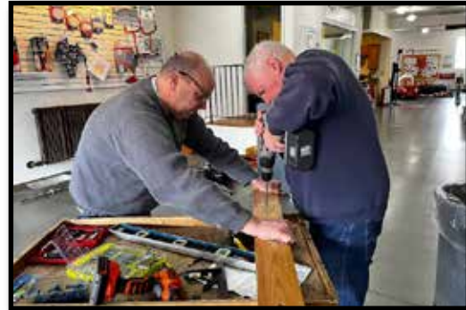
Larry Gordon & Tony Caruso Do Some Prep Work to Hang Boards
