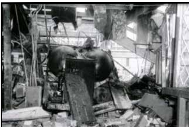
Double tank truck inside garage
