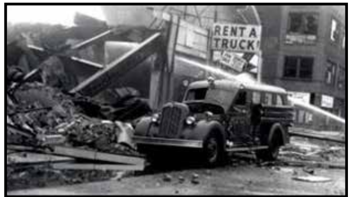
Engine 28's damaged pumper in front of building
