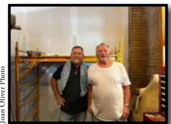
Pete Corso & Jerry Betram work on firewall
