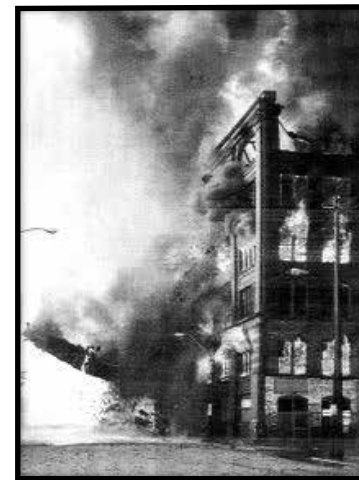
One of the walls collapsing
